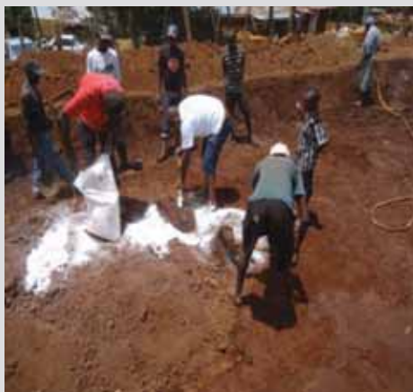
Mixing soil with lime (left). Preparing mud for plastering (right).
