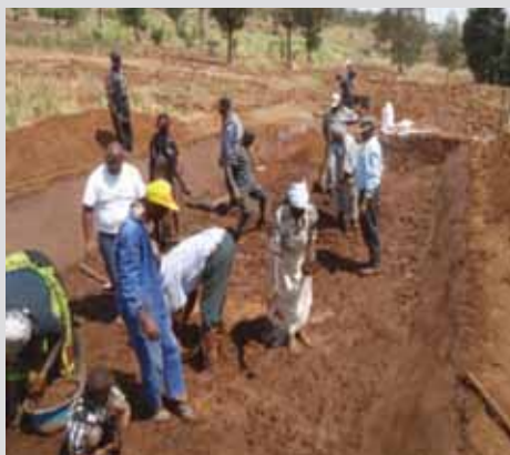
Mud is spread (left), a thin mud paste is smeared and water added to avoid cracking (right).
