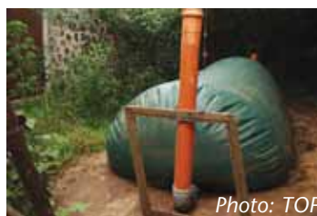
The flexi gas biogas (above) system is housed in a greenhouse to protect it from the sun and prolong its lifespan(below)
