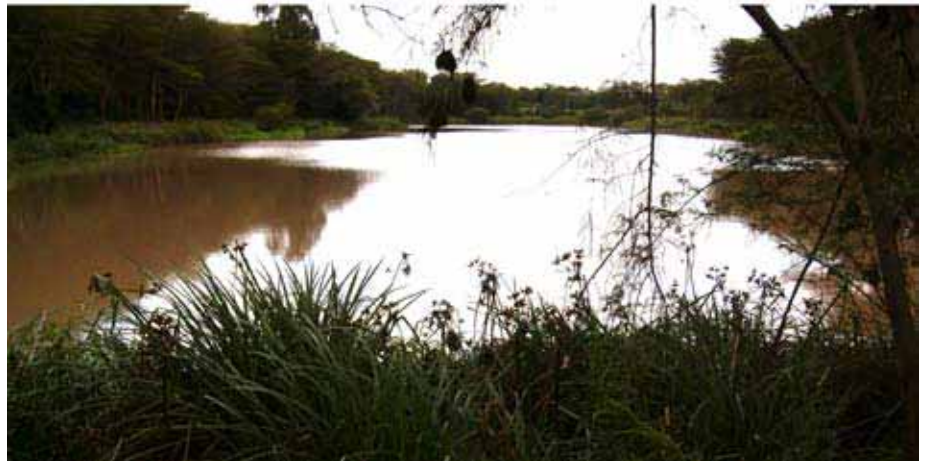
The Naishi dam (above). Farmer Elishiba Wanjiku (below) draws water from her home dam.
