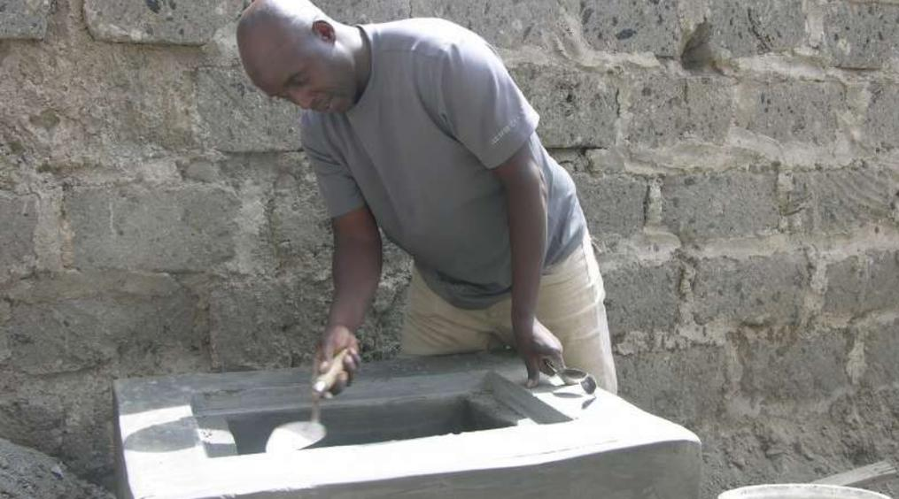
Mr Solomon Njuguna demonstrates how to build a biogas biodigester
